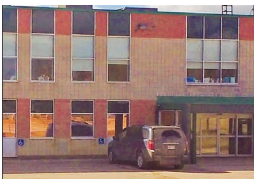
The Grand Valley and District Community Centre was evacuated Sunday, March 19, after a carbon monoxide leak was detected. Emergency response teams from the Grand Valley and District Fire Service, Orangeville Fire Service, Dufferin County Paramedics and the Ontario Provincial Police were on site providing assistance. Several people were transported to hospital. PHOTO BY MARNI WALSH
