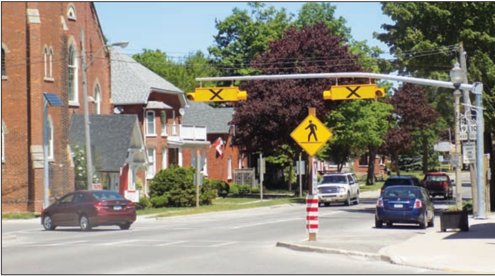
The recently installed Crosswalk located at Hwy 89 and William Street will be replacing the Courteously Crossing that was previously located at this intersection. John Telfer, CAO at the Town of Shelburne tells the Free Press that the new Crosswalk is being inspected by the MTO and should be fully functioning by Thursday of this week. PHOTO BY MICHELLE JANZEN
